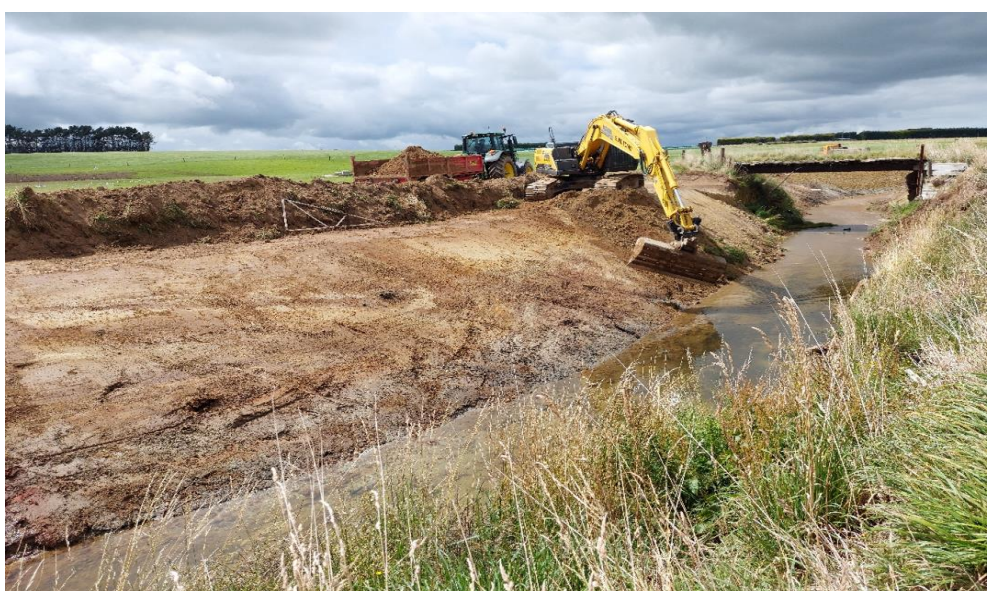
Photo below highlighting a 2:1 batter construction on McSwag property
