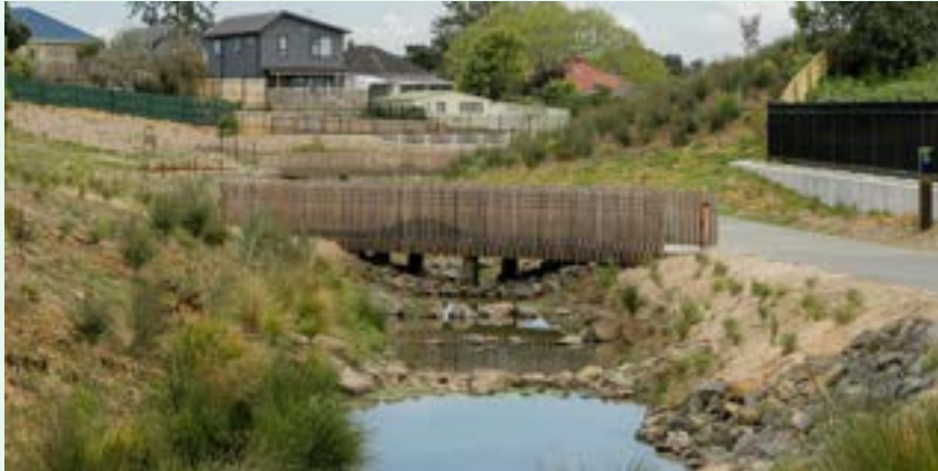
Te Auaunga, Oakley Creek. Photo: Kāinga Ora
