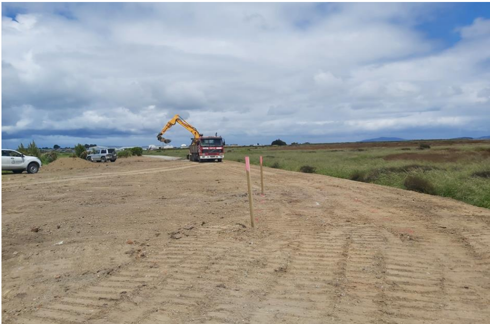
New walkway construction behind Stabicraft
