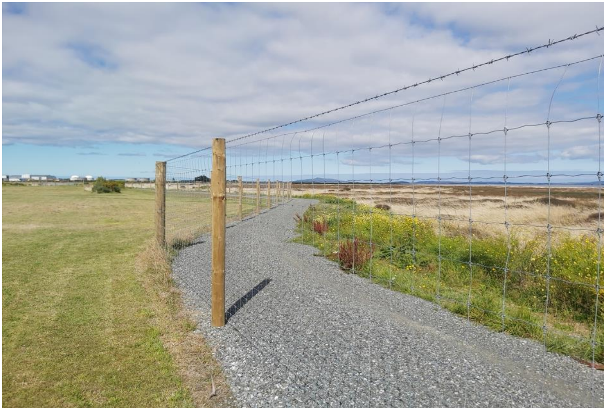
New walkway and security fences behind Stabicraft
