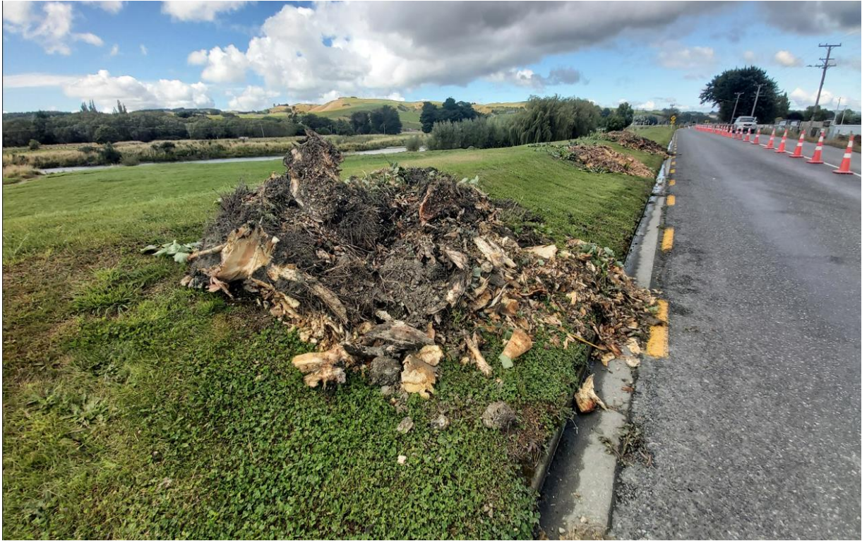
Results from stump borer and pick, before tree roots removed
