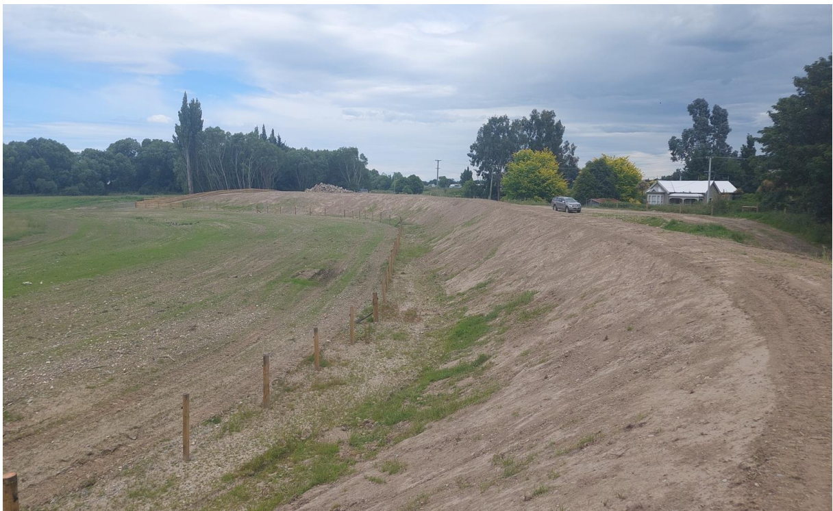
Ontario street bank completed
