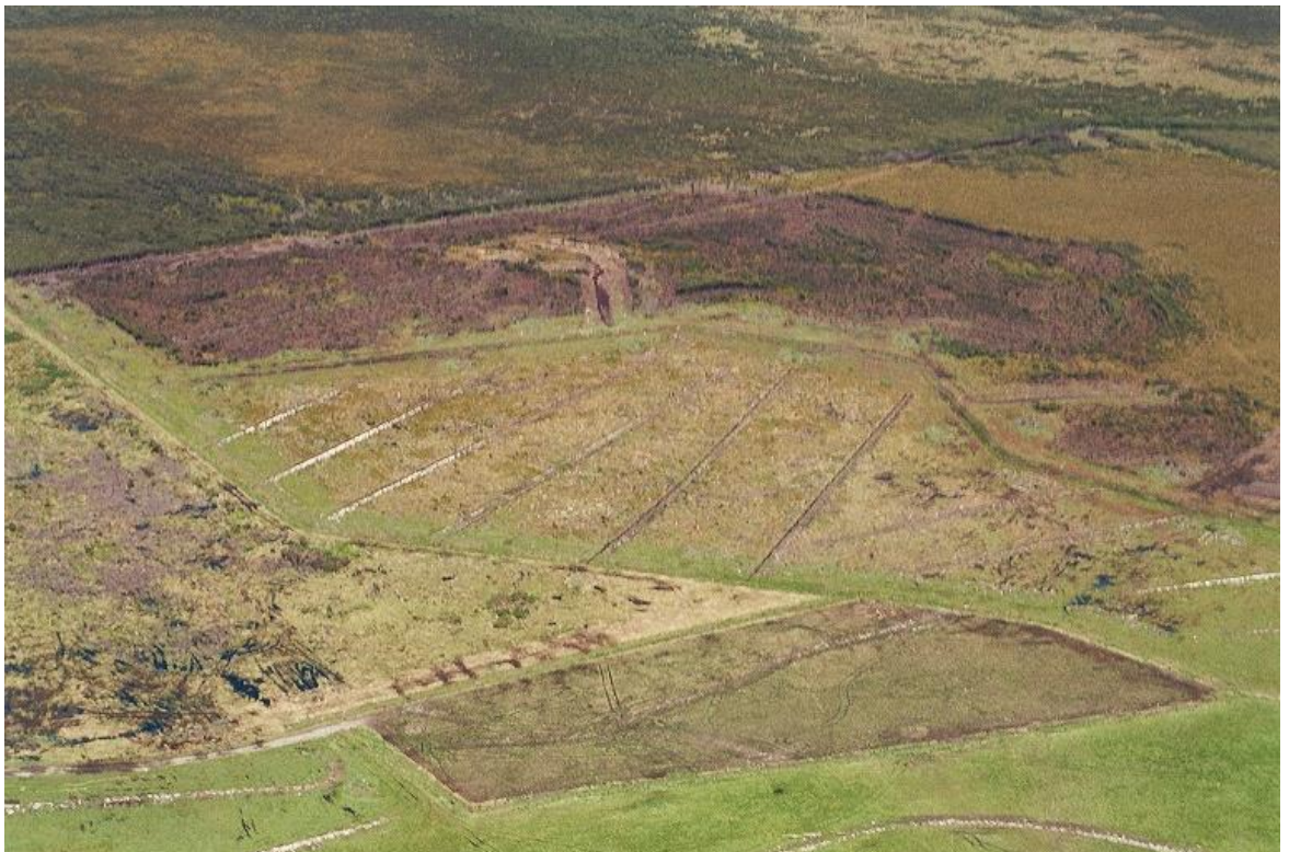
Drainage works on the margin of the Awarua Ramsar Wetland of International Importance
