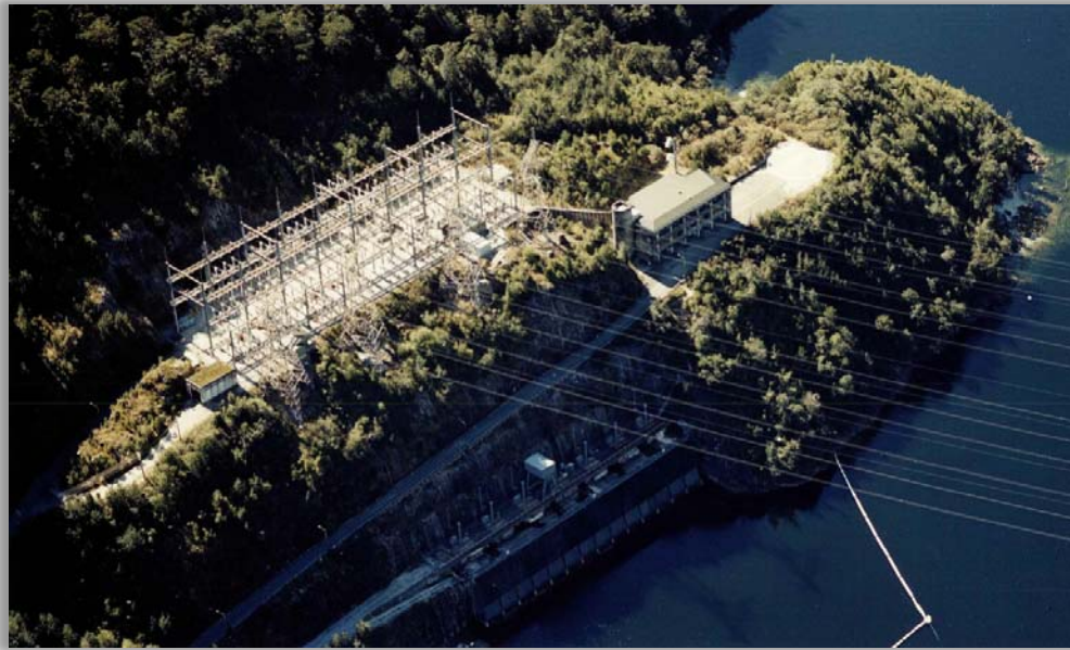
Image 1 – Manapouri Power Station – West Arm Lake Manapouri
