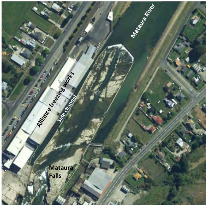
Figure 3-3 Matura River at Alliance freezing works site
