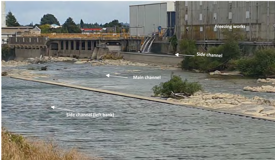
Figure 3-5 Maitara River channels at Alliance freezing works site
