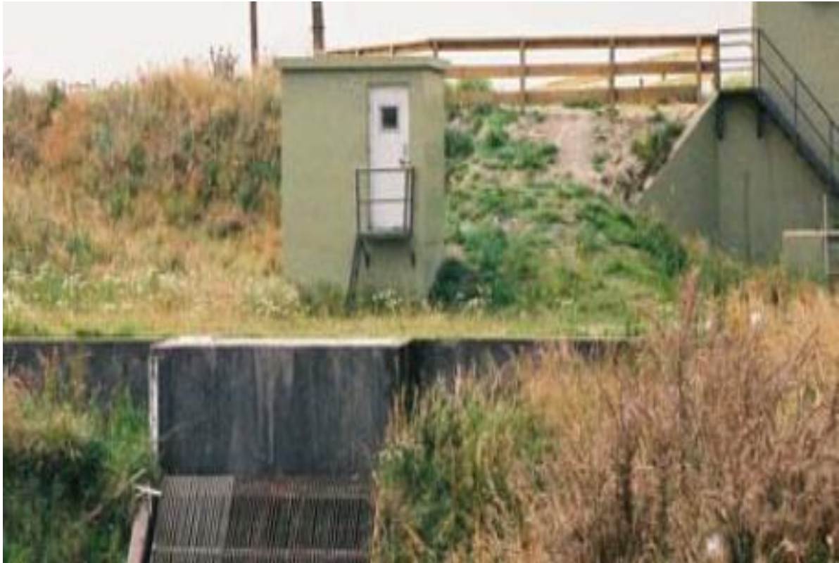
Figure 12: View of intake structure.
