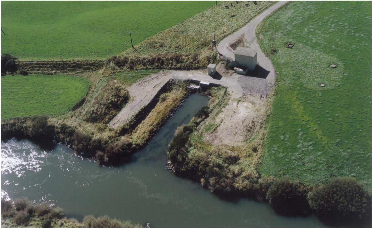
Figure 2: View of the Alliance water take from the Oreti River.
