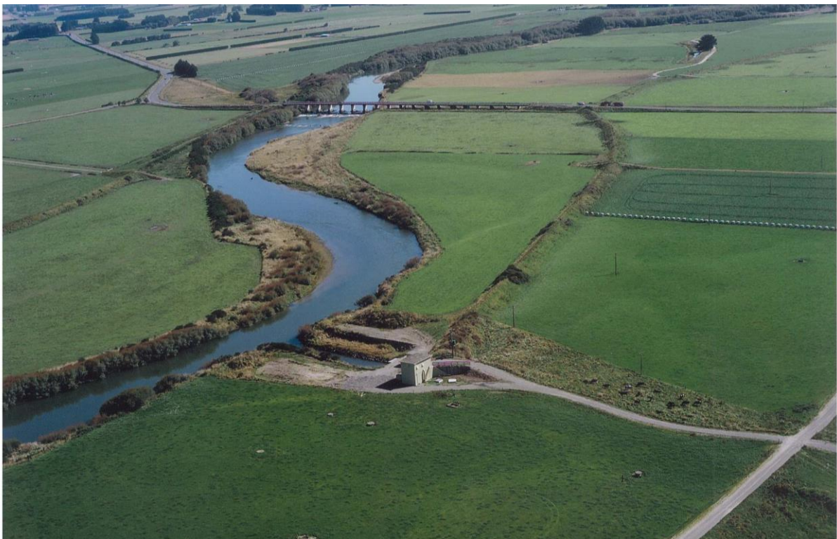
Figure 3: View of the Alliance water take and Wallacetown Highway Bridge.
