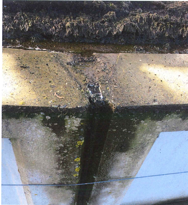
Typical overflow down joint from overfull pond at low side of the pond. Grout infill and sealant are all in good condition.
