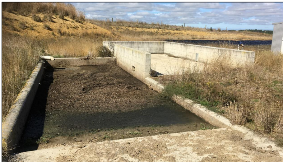
Figure 3: Large stone trap adjacent the effluent pond
