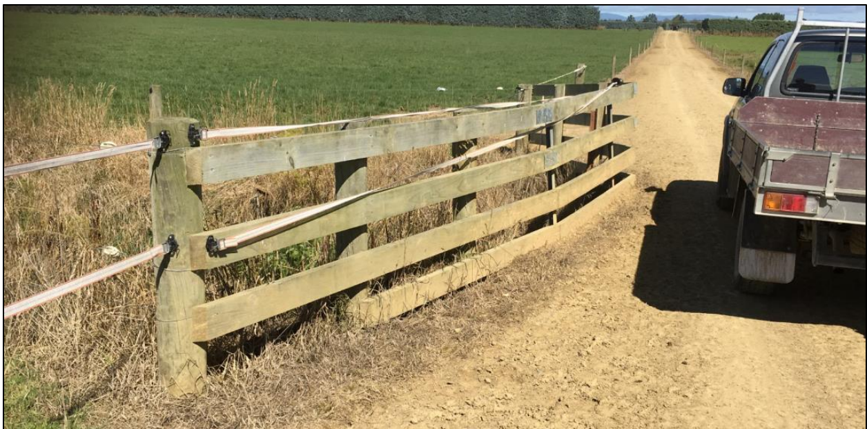
Figure 18: Laneway crossing with kickboard to prevent direct runoff into creek
