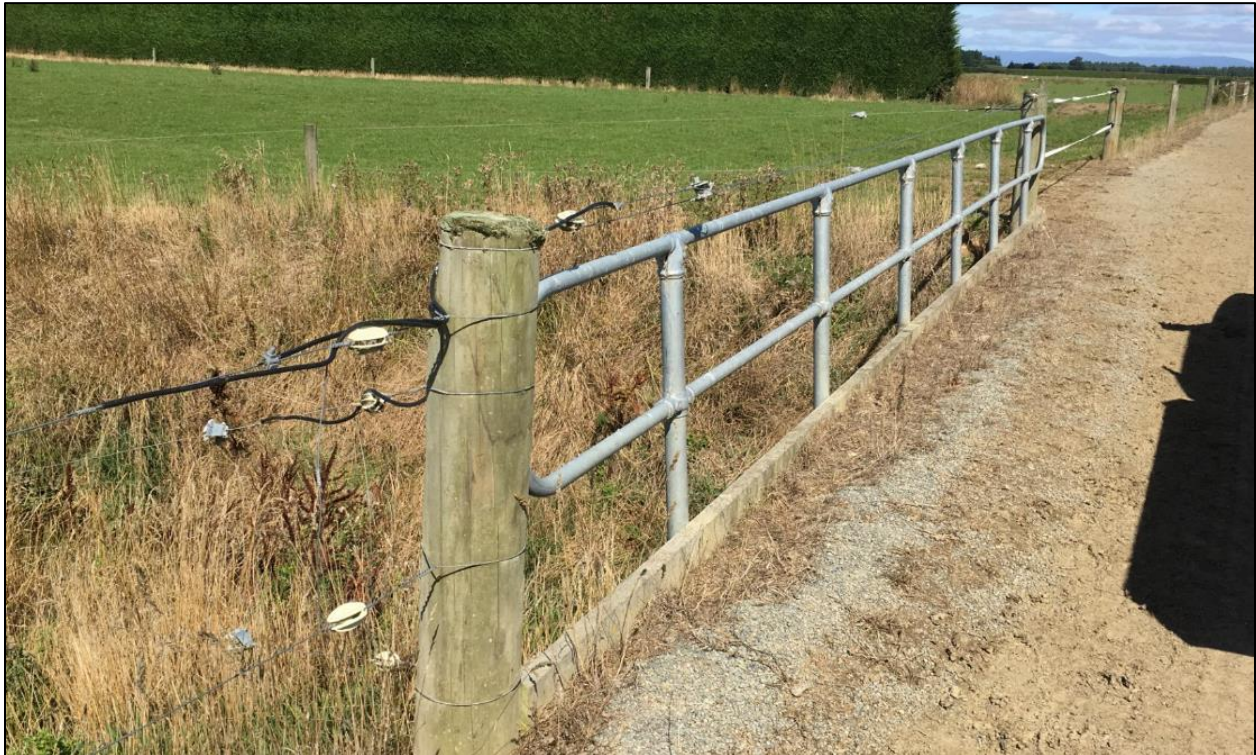
Figure 19: Laneway crossing with kickboard to prevent direct runoff into creek
