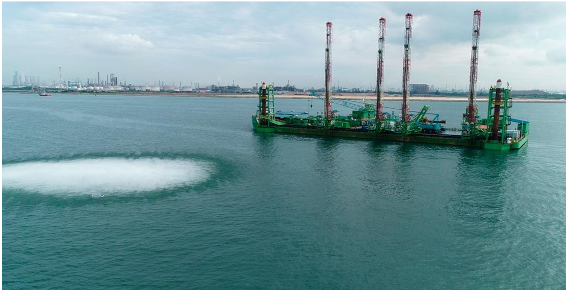
Figure 14: Water boil effect from underwater blasting (indicative only)
