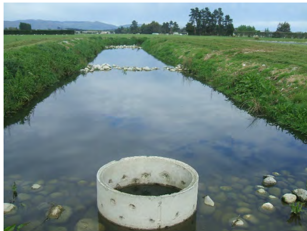
Figure 3-3: Soakage channel and outlet
