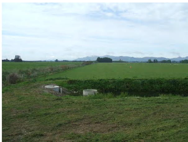
Figure 3-4: Soakage channel and discharge structure showing the Meadow Burn (on left)
