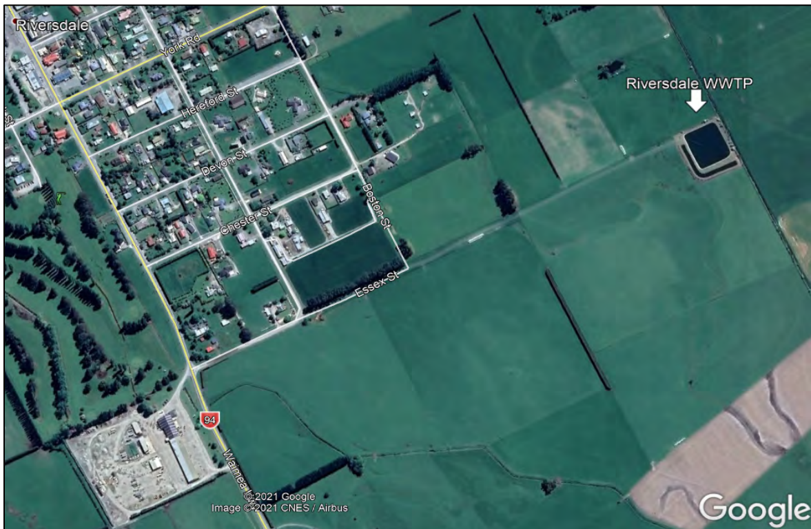
Figure 1: The Riversdale Wastewater Treatment Plant
