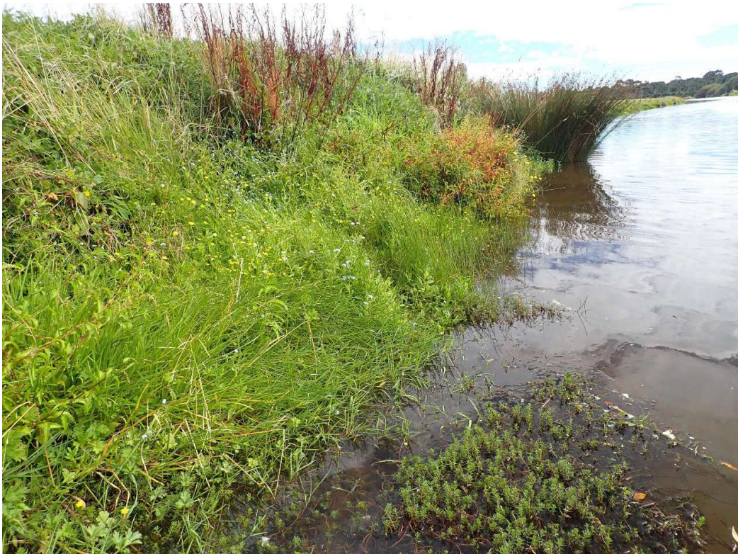
Photograph 4: (WP 050 Unsuitable – Steep Banks)
