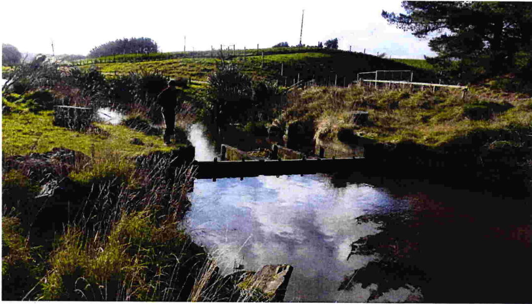
PHOTO 2: VIEW OF THE TIDAL GATES LOOKING UPSTREAM
