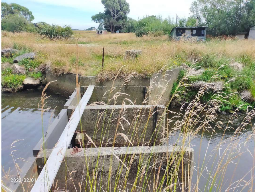
Photograph 29: Titiroa Tide Gates closed
