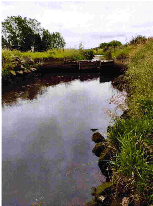
Photo 1: Titiroa Tide Gate Structure Opening, view upstream.
