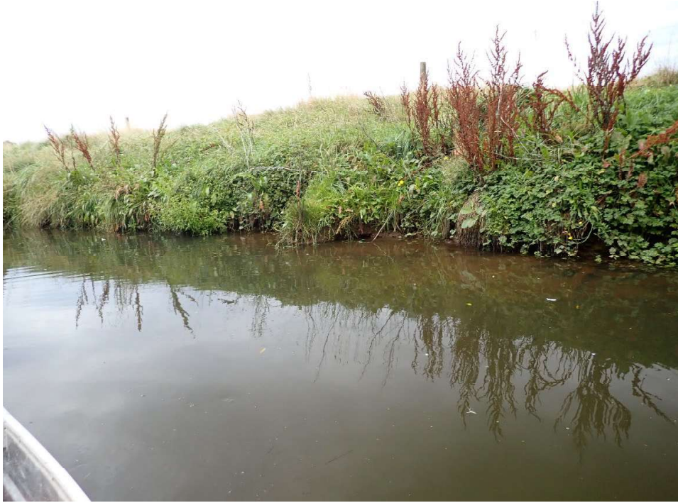
Photograph 7: (WP 034 Unsuitable, example of vertical bank)
