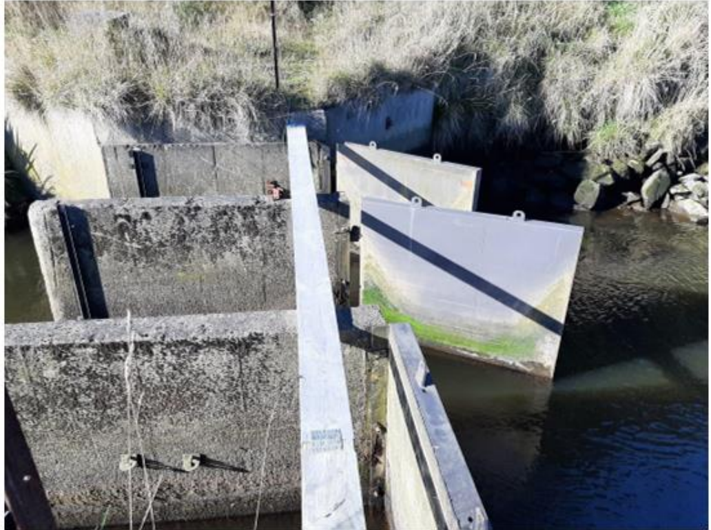
Figure 2 – tide gate structure – partially closed on a rising tide.
