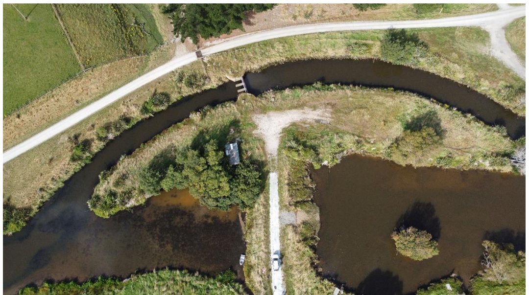
Figure A2: Titiroa tide gates – drone view of closed gates and diversion channel.
