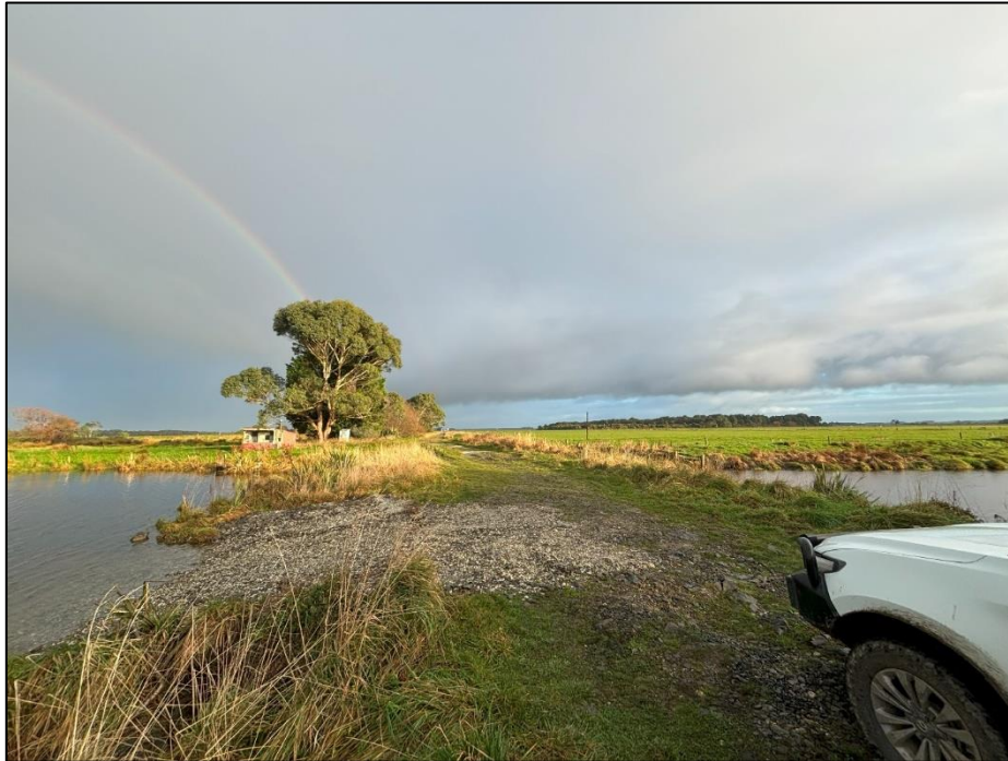
Figure 1-3 – Photo of spillway taken on the 2 nd July 2024
