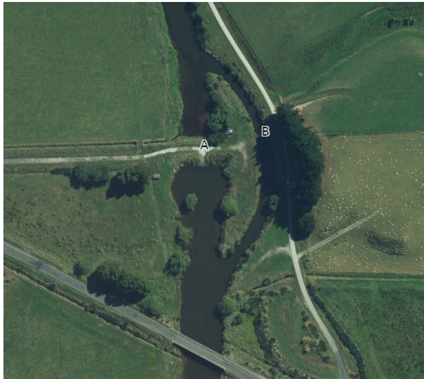
Figure 1 The Titiroa tide gates, diversion and dam/weir
