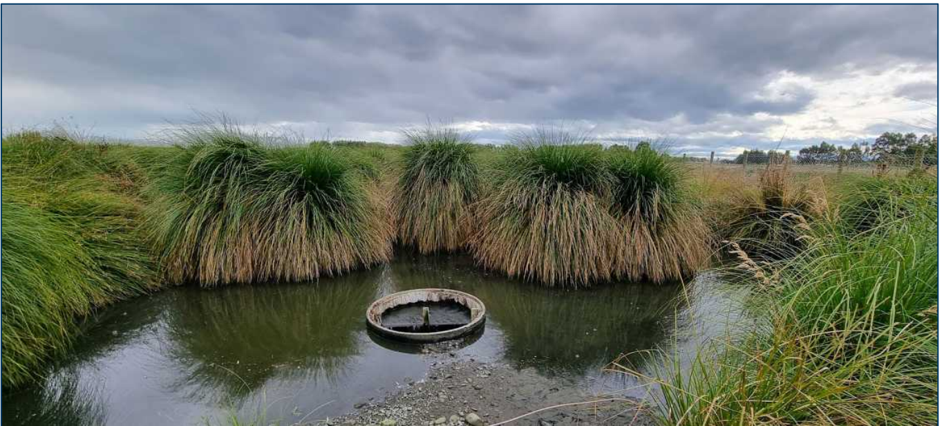
Figure 7 Wetland cell drainage point
