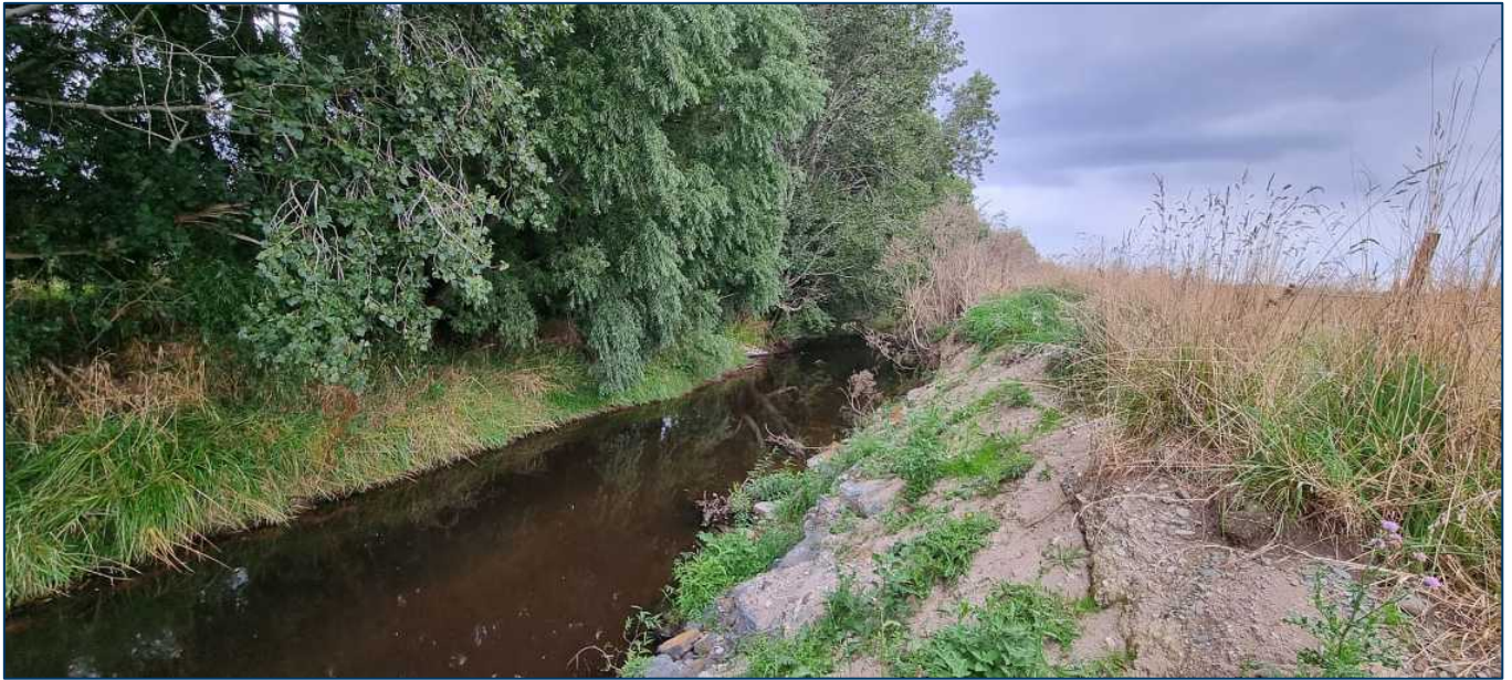
Figure 22 Downstream of diffuser
