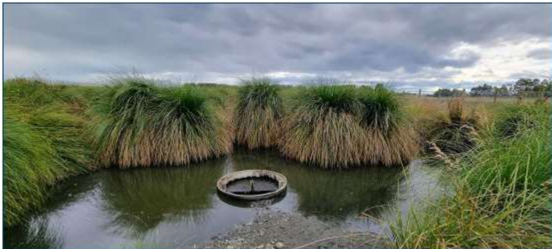
Wetland cell drainage point
