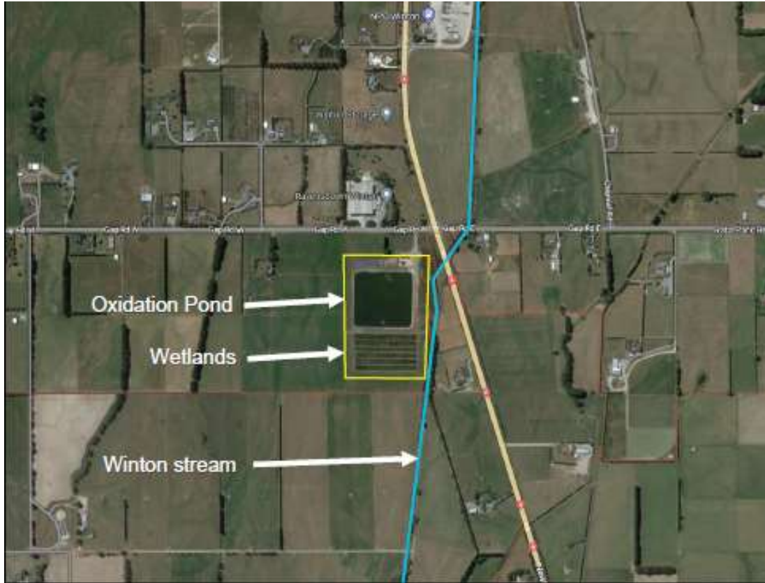
Winton WWTP (yellow outline) and Winton Stream (blue line)
