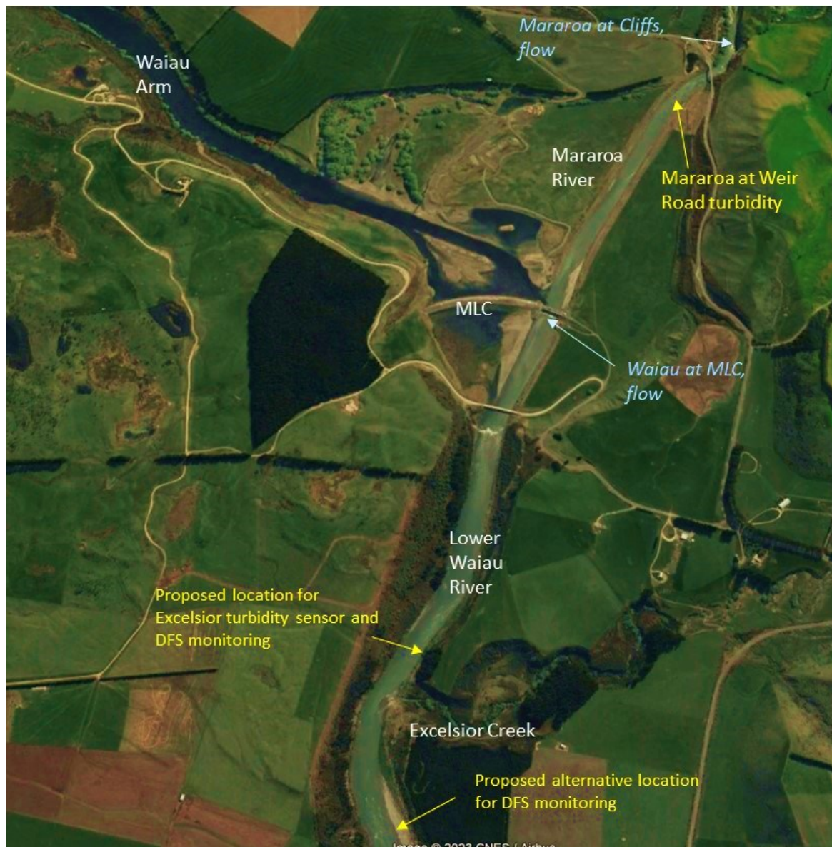
Figure 5.5: Location of turbidity and flow recorders to be used in the monitoring programme for the duration of the excavation works (Source: Appendix D).
