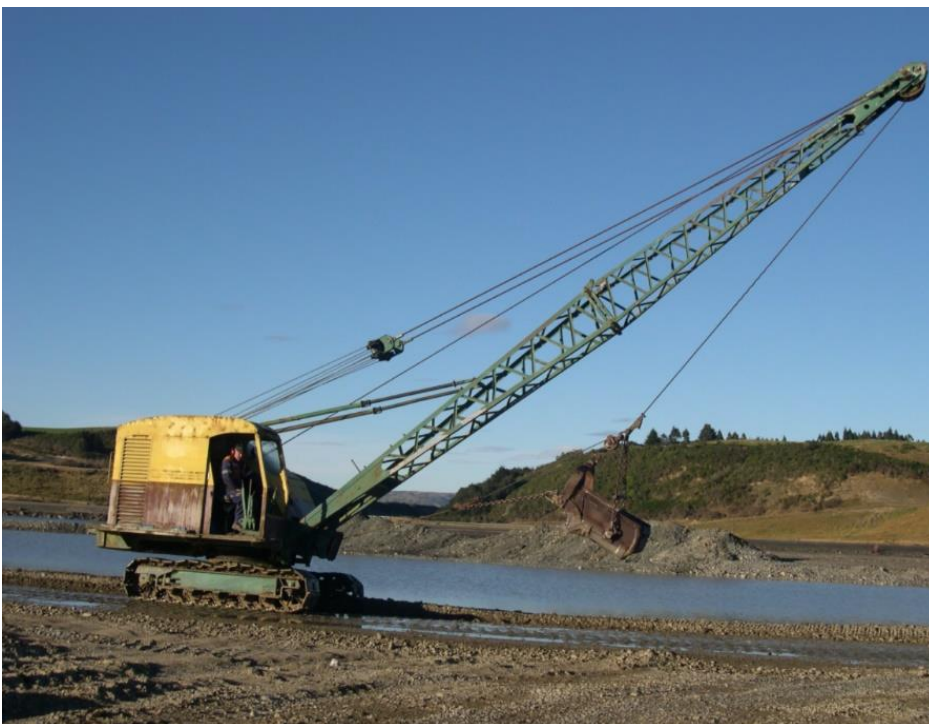
Figure A.2: Small dragline setup used in 2007 Waiau Arm excavation
