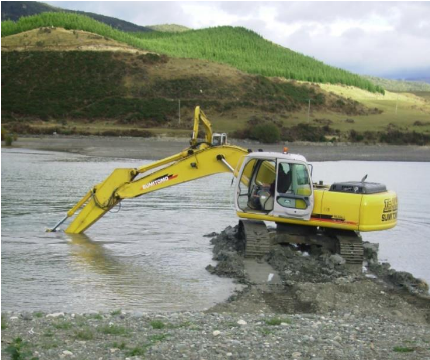
Figure A.3: Excavator working from bund in 2007 Waiau Arm excavation
