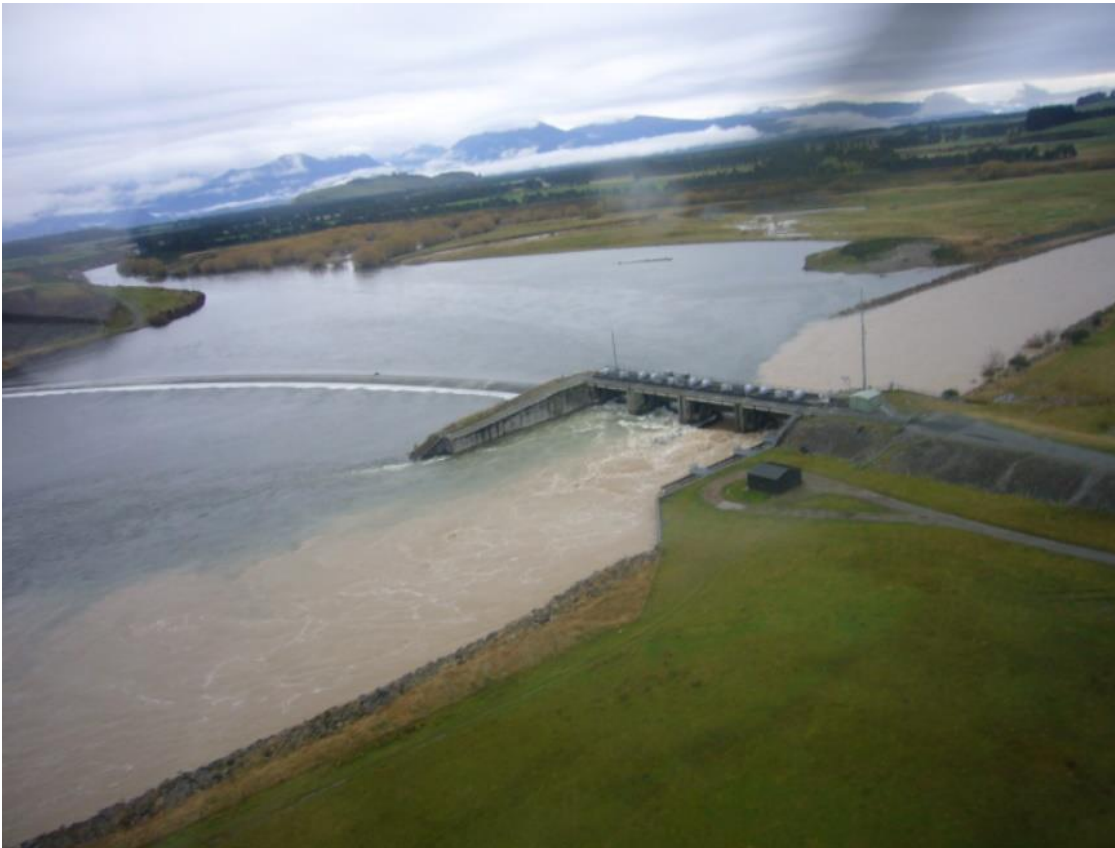
Figure 3.2: Floodwater spilling over MLC weir, 27 April 2010, approximate flow 800 m 3 /s (following a flood peak of 1130 m 3 /s on 26/4/10).
