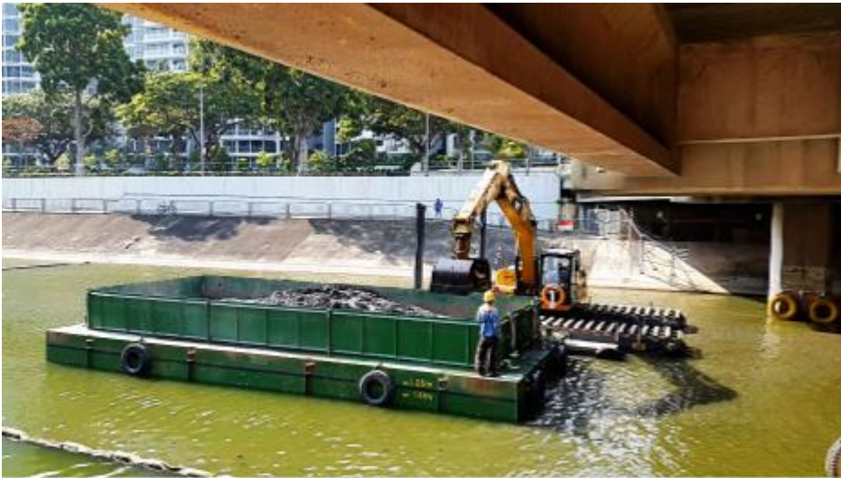
Figure A.4: Excavator working from floating platform with hopper barge
