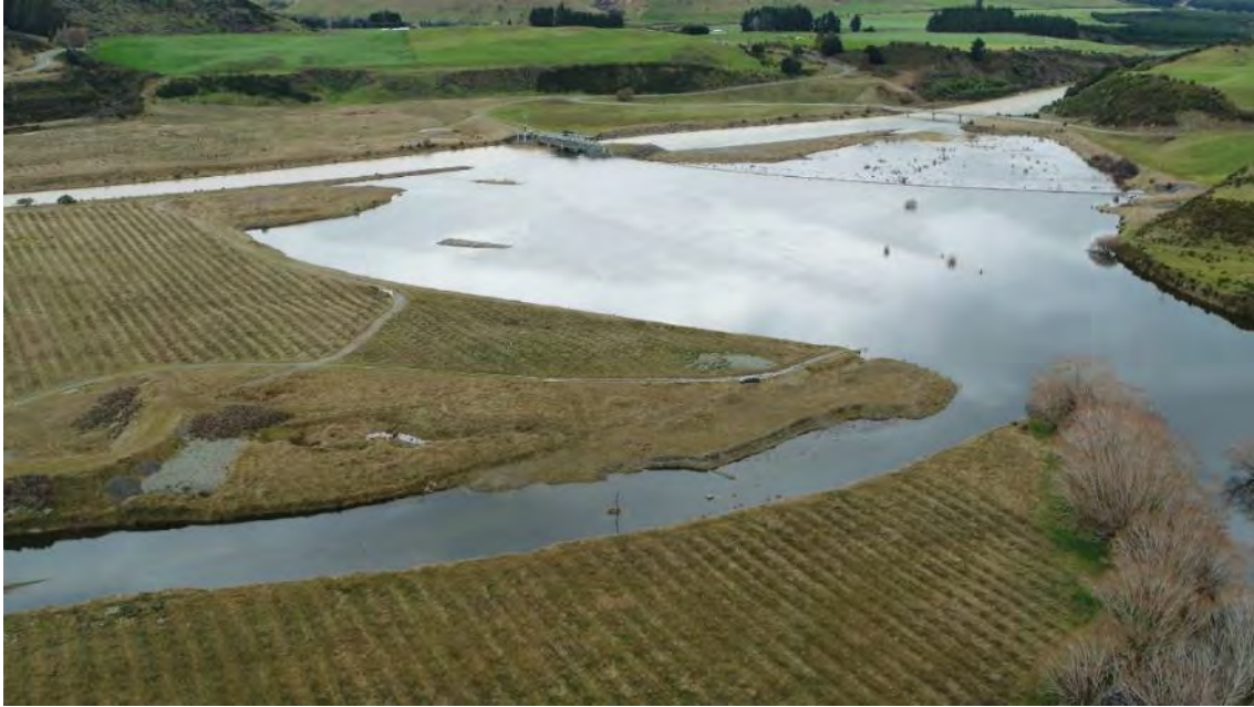
Photo 1: Manapōuri Lake Control and Waiau Arm during high lake levels, looking downstream. The Mararoa River (channelised) is visible top left. Figure provided by Meridian / Nick Key.
