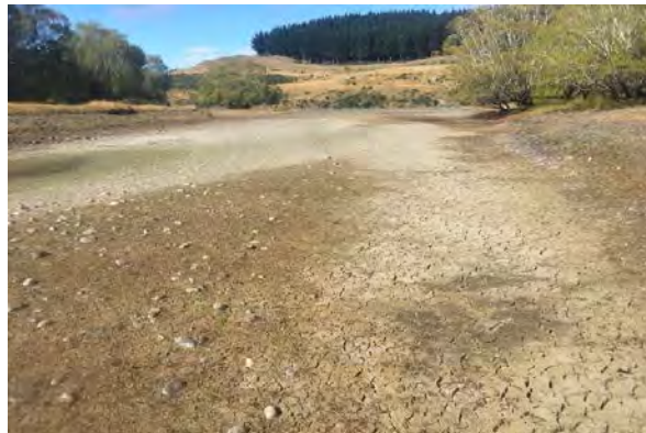
Channel 2 dry during low lake levels.
