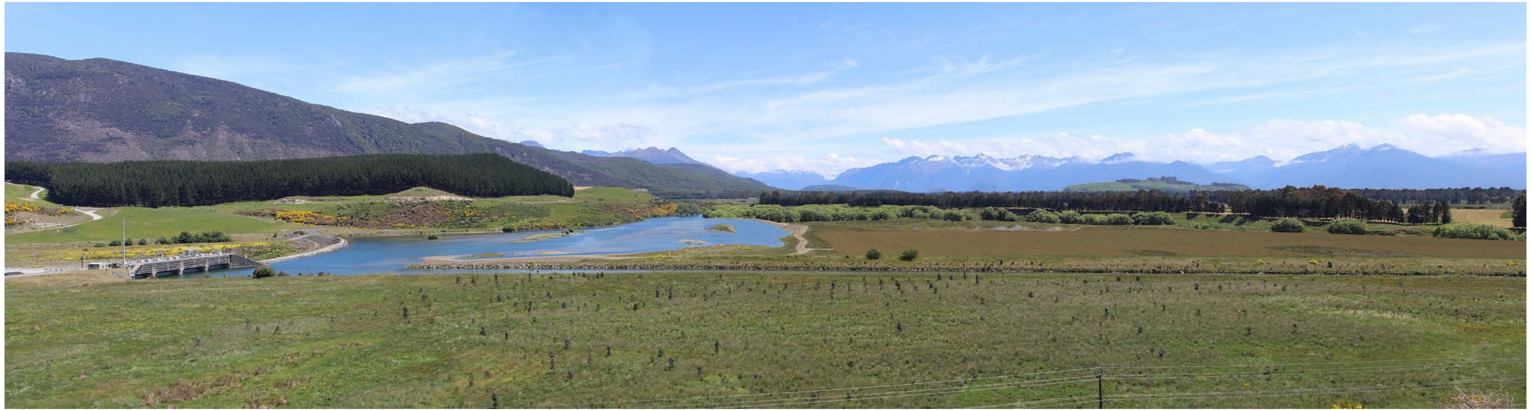
Visual Simulation 1E - 3: After construction when water level is the same as the day of site visit (177.9m).
