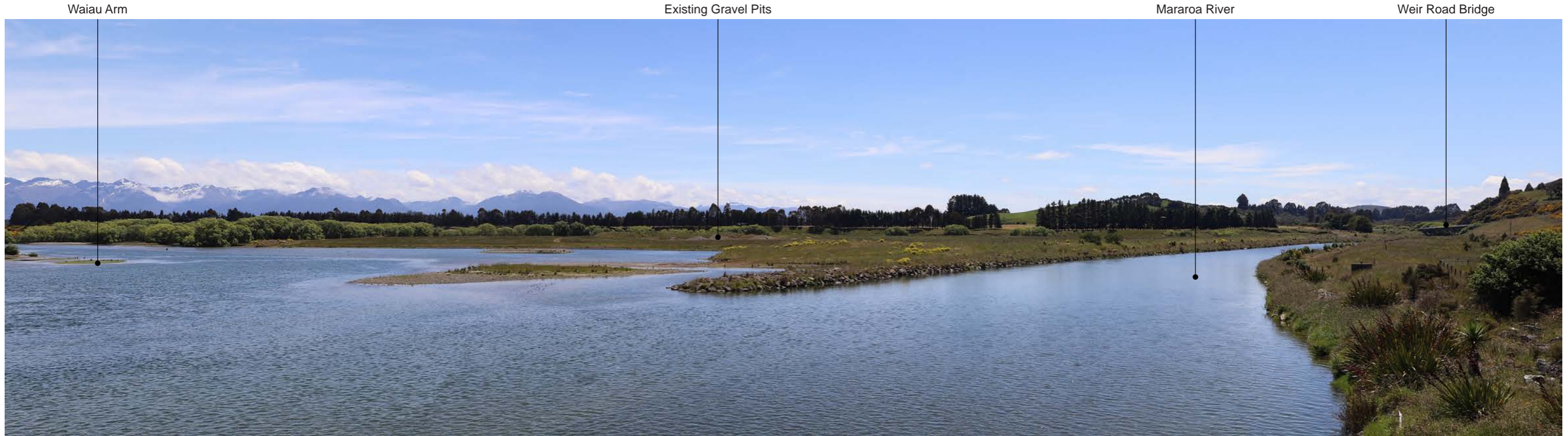
Site Appraisal Photograph C: View looking north from the Manapouri Lake Control structure.
