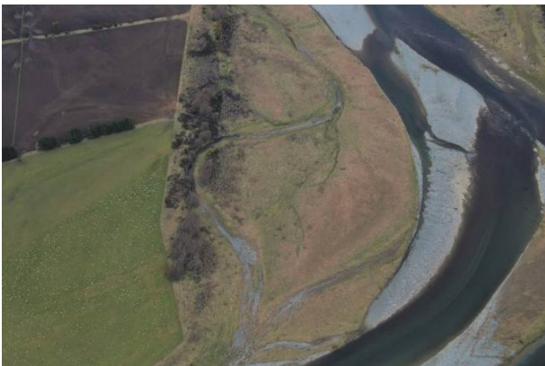
Figure 13: Redcliff Side Braid Wetland
