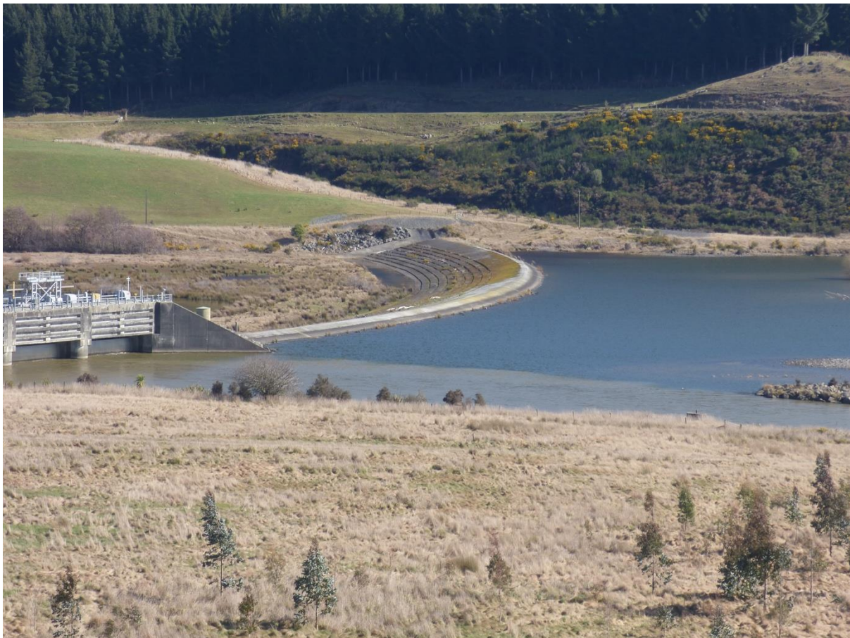
Figure 1 The MLC and turbid water from the Mararoa being diverted into the Lower Waiau River. 31 August 2024.
