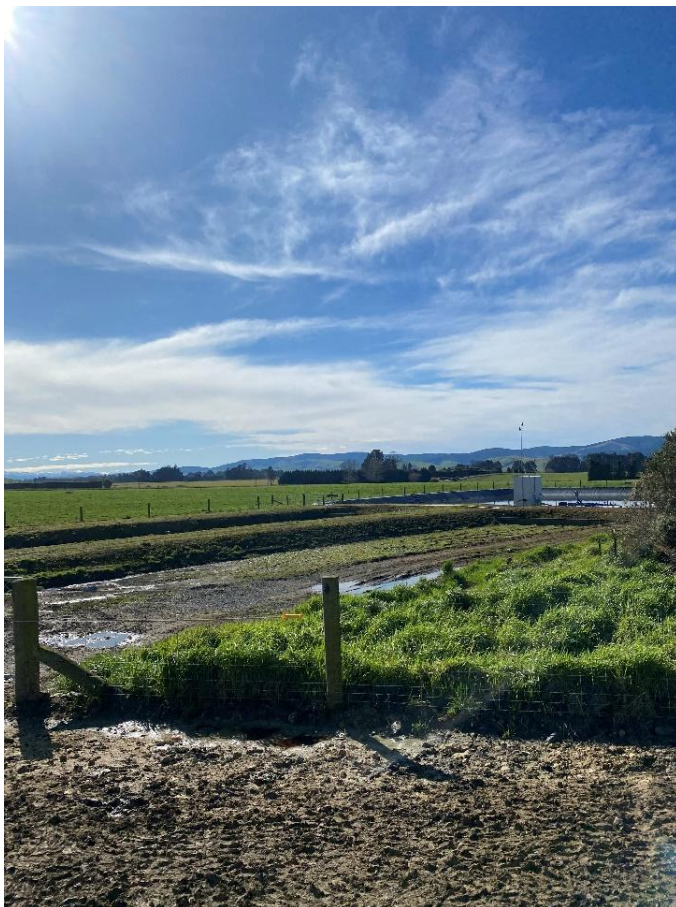
Figure 6: Photos of x2 sludge beds and lined pond in background, Landpro, 27/08/2024.
